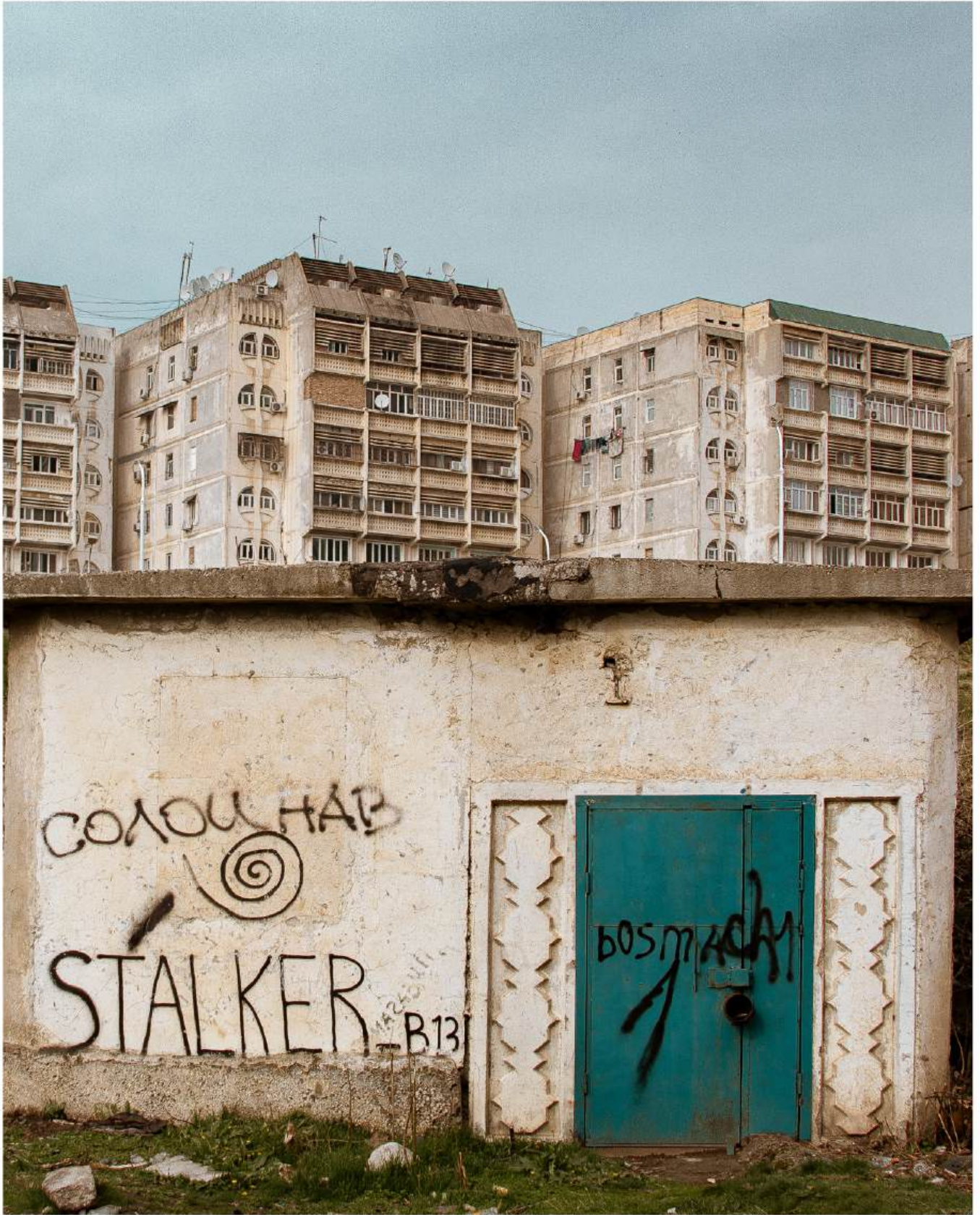
Panel Housing Blocks | 22/7 Zarafshon Street
